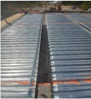
Figure 1: 2 Layers of roofing felt placed in link slab zone to prevent bond between the deck and girder.
