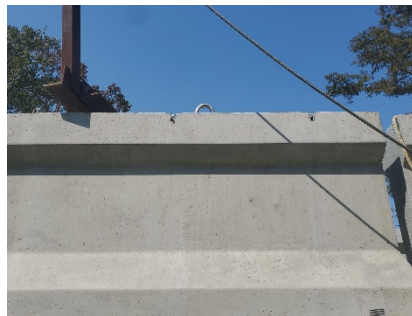
Figure 2: Top of Girder Flange is not raked. SIP Angles are not welded to girders, but instead utilize a metal strap for support.
