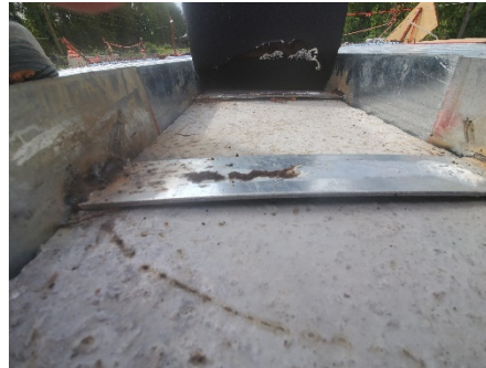
Figure 2: Top of Girder Flange is not raked. SIP Angles are not welded to girders, but instead utilize a metal strap for support.
